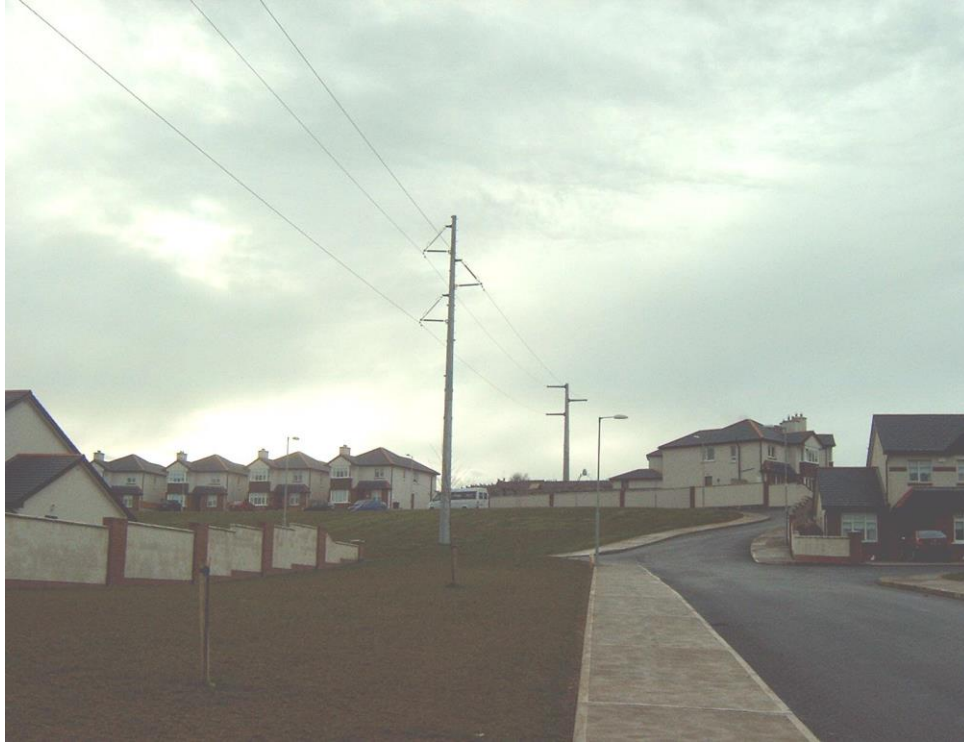
Figure 14: 110 kV Monopole Overhead Line in Cork
