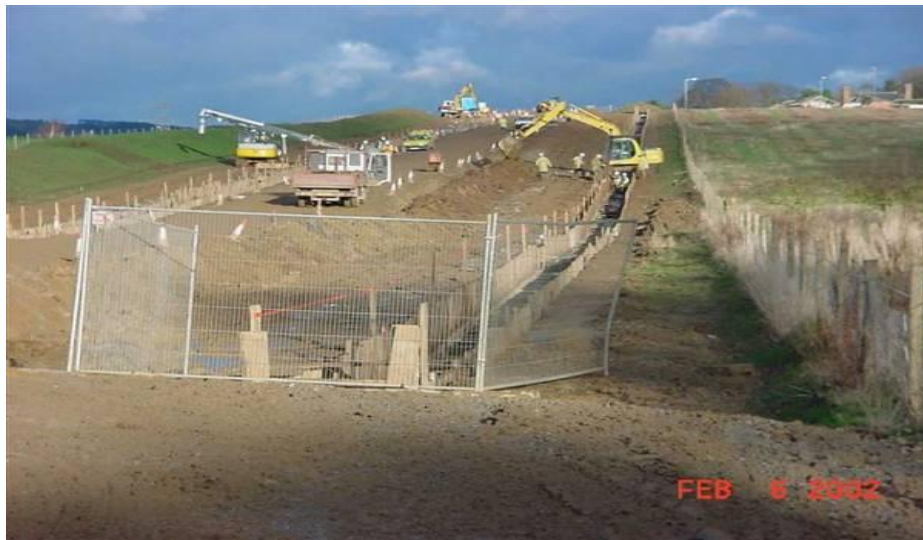
Figure 8: Photographs of a 400 kV Double Circuit Cable Being Installed Cross-Country
