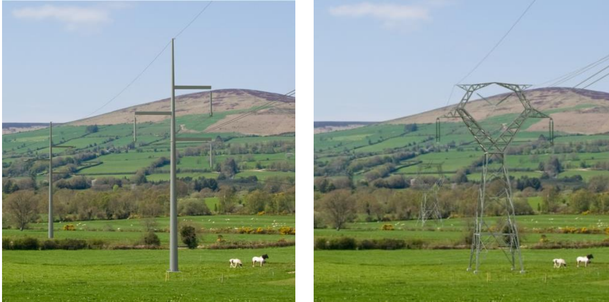
Figure 164: 'Atkins' Monopole Design and Proposed IVI Lattice Tower
