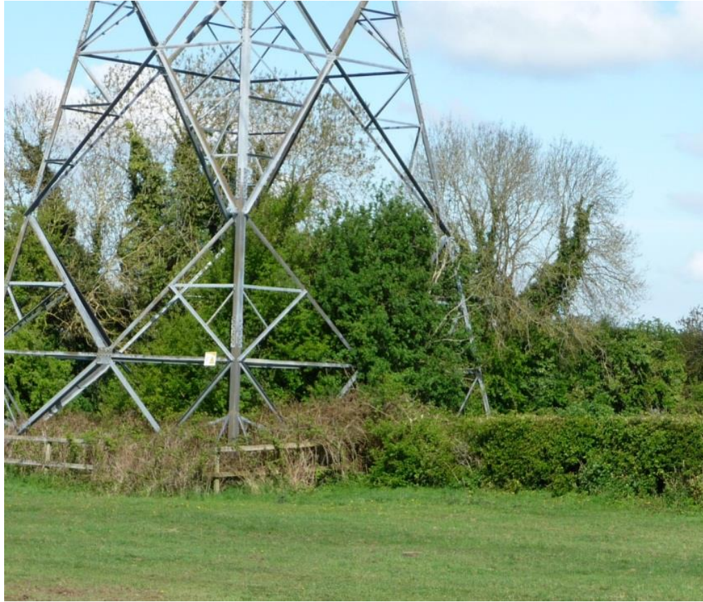
Figure 9: Photograph of a Tower Straddling a Hedgerow with Vegetation Re-established
