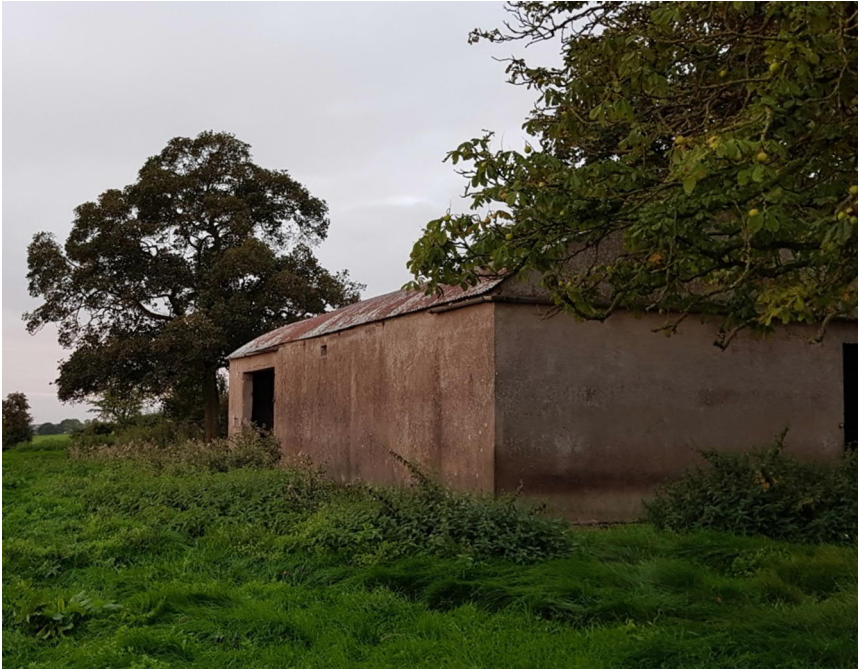
Photograph 3: Tin-roofed shed at substation site.
