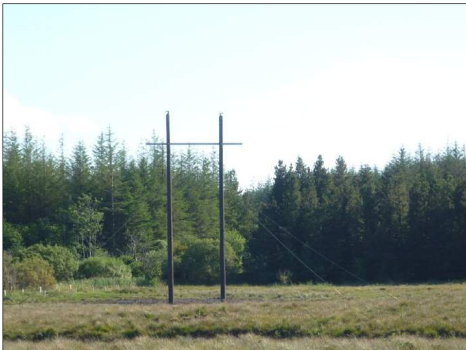
Stay lines in place, Donegal 110 kV Project
