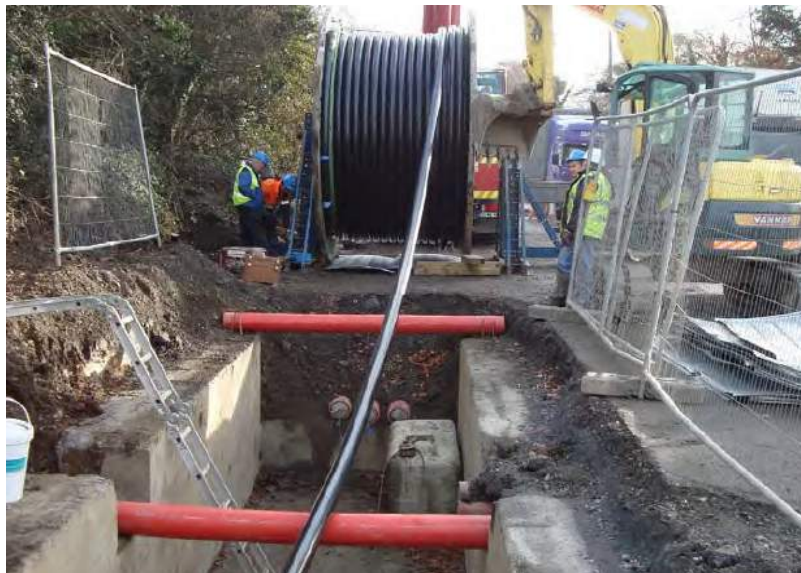
Typical HV Cable Installation
