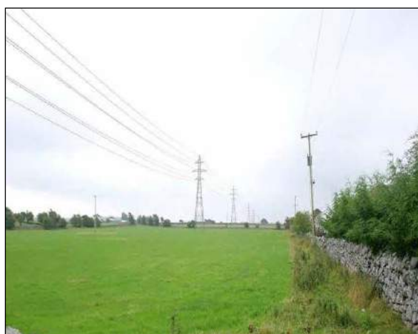
Typical 110 kV double circuit structures
