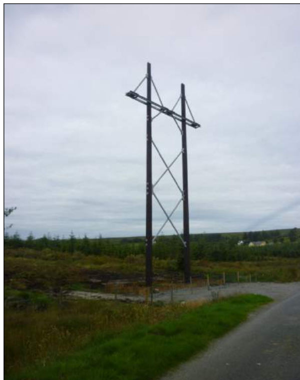
Braced double wood poleset
