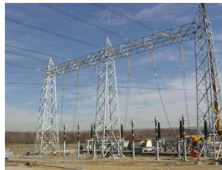
Figure 5: Overhead line cables transition station (400kV)
