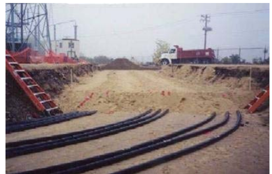
Figure 18: Installation of 400 kV XLPE cables
