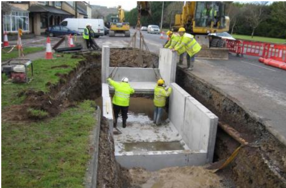
Figure 2-11: Typical joint bay under construction (pre-cast)
