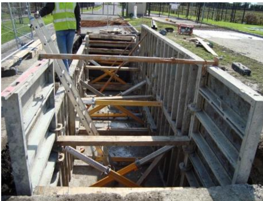
Figure 2-9: Typical joint bay under construction (in-situ)
